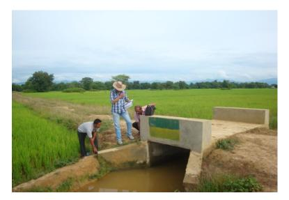
3. Boulder Bank Pitching with Hume Pipe at Holowguri (Borhula), Borhula MWS : The size of the Hume pipe culvert looks less than required for the width of the drainage line, two rows of hume pipe would have been adequate . Boulder pitching is done without wire crate as mentioned in the estimate. The work was not finished completely.
