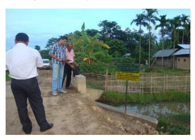
7. **Agri Field Bund at Padumpukhuri village, Padumpukhuri MWS** : The Agri field bund work was not finished. It was advised to complete the work by maintaining the side slope and the depth of filling.
