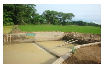
**2. Nalla Bund with Slab Culvert at Amguri No.1 village, Amguri MWS** : The objective of the slab culvert as well as the Nalla Bund is fulfilled as it is allowing excess water to pass through it easily. The quality of the construction looks good. The work was not finished completely.
