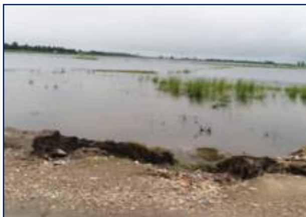
Figure 8: River Bank Erosion
